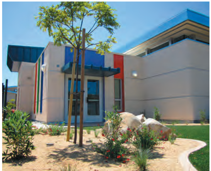
Morse High School Child Development Center. Design included drought tolerant, low maintenance plant materials and one of the San Diego Union School Districts first drip irrigation systems.
